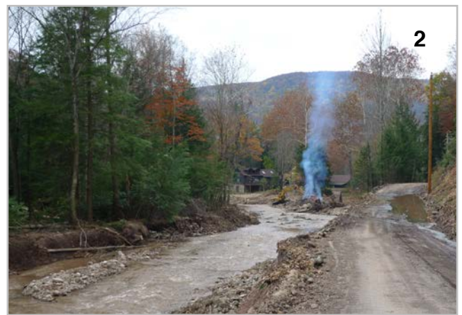
2. Snagging and burning of woody debris, gravel, realignment of channel, and installation of rock veins. (mid to late September, 2011)
