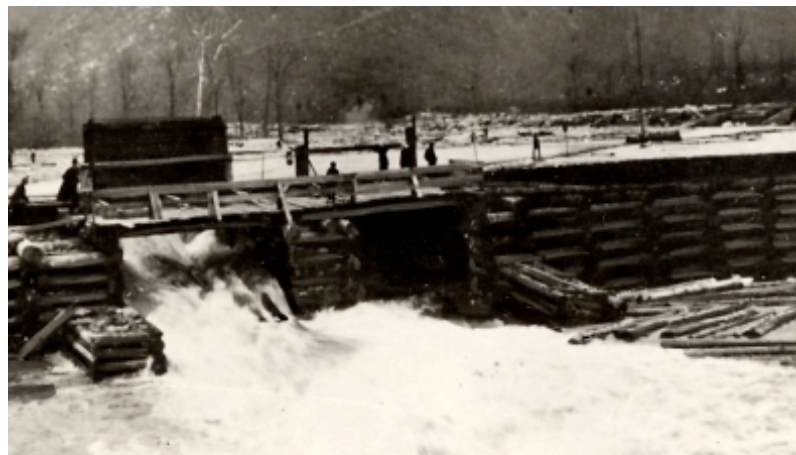
During the peak of the logging boom in the 1880s, watersheds such as this one - Pine Creek in the West Branch of the Susquehanna River - were completely denuded; their hillslopes were stripped bare of protective forests. Stream channels were straightened, snags removed, and temporary “splash dams” constructed to float the logs downstream to the saw mills and log booms of the Susquehanna. As a result, millions of tons of sediment were washed into the rivers, destabilizing the streams for decades. Geomorphic and hydrologic studies are showing that over the past 100 years, these logging legacy sediments are being flushed downstream with each major flood.
