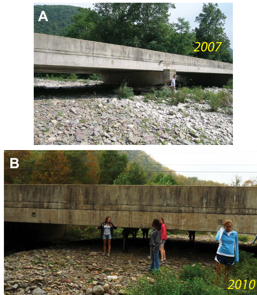
Figure 31. Ground view of aggradation at Highway 14 bridge at Roaring Branch. Several meters of remobilized logging legacy gravel had to be removed from under the bridge several times in the past 20 yr. (A) View in July 2007. (B) View in October 2010, showing ~1 m of aggradation in 4 yr.
