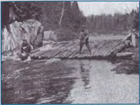
Figure 7. Log apron built across bedrock constriction, to prevent log jams at the waterfall.
