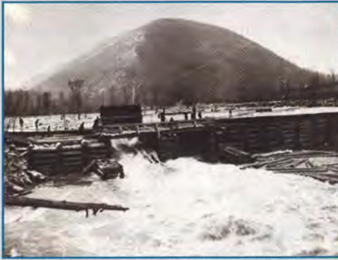
Figure 8. Sluicing logs through the gate of Flooks Run Splash Dam on Little Pine Creek in Lycoming County, Pennsylvania (Forest Leaves, published by the Pennsylvania Forestry Association, vol. 17, no. 12, pg. 185, (December 1920). Note the clearcut hillslopes.
