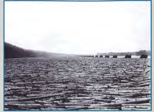
Figure 9. Susquehanna log boom and crib structures at Williamsport, PA.
